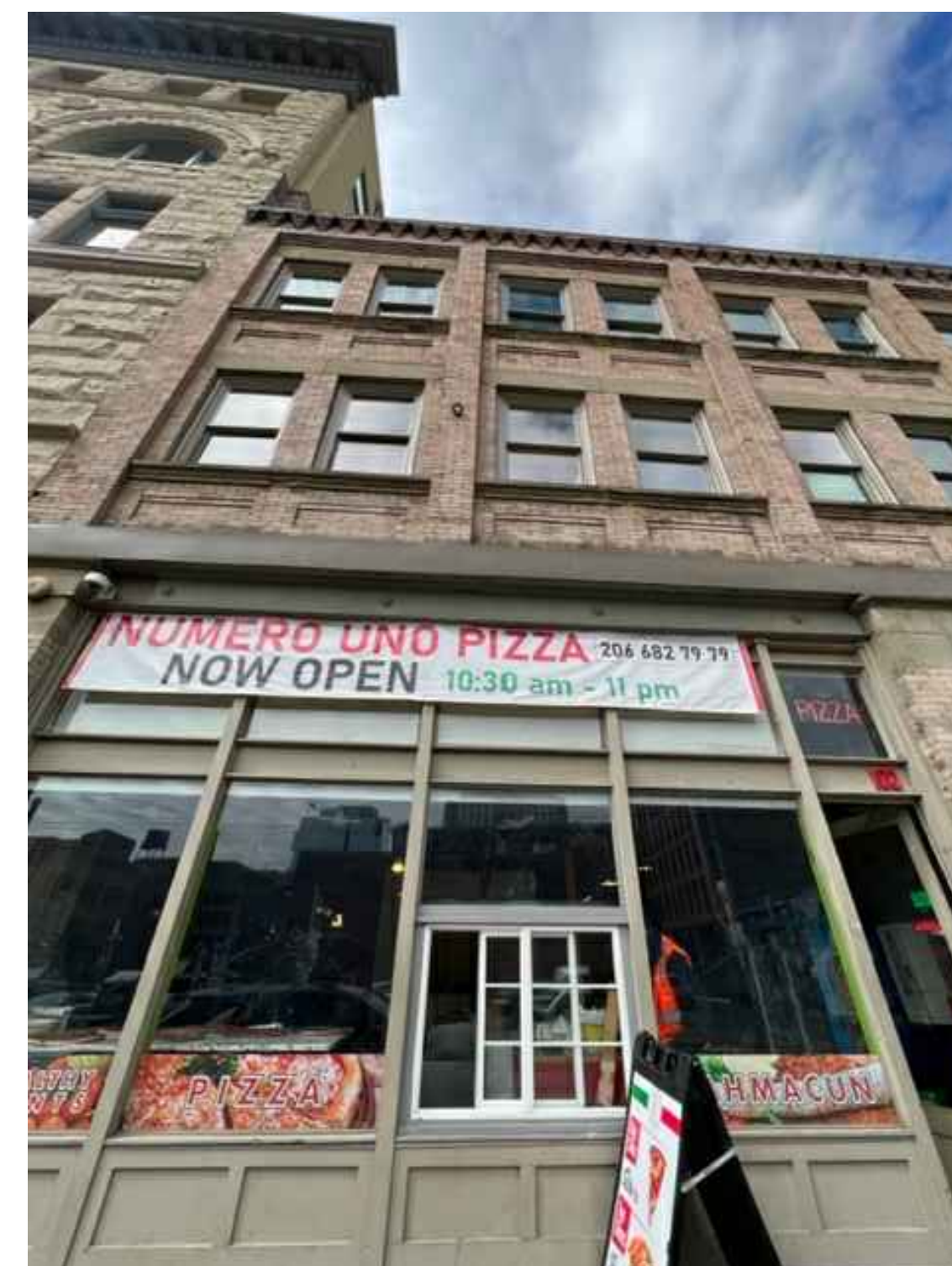
view of existing signage & servery window
