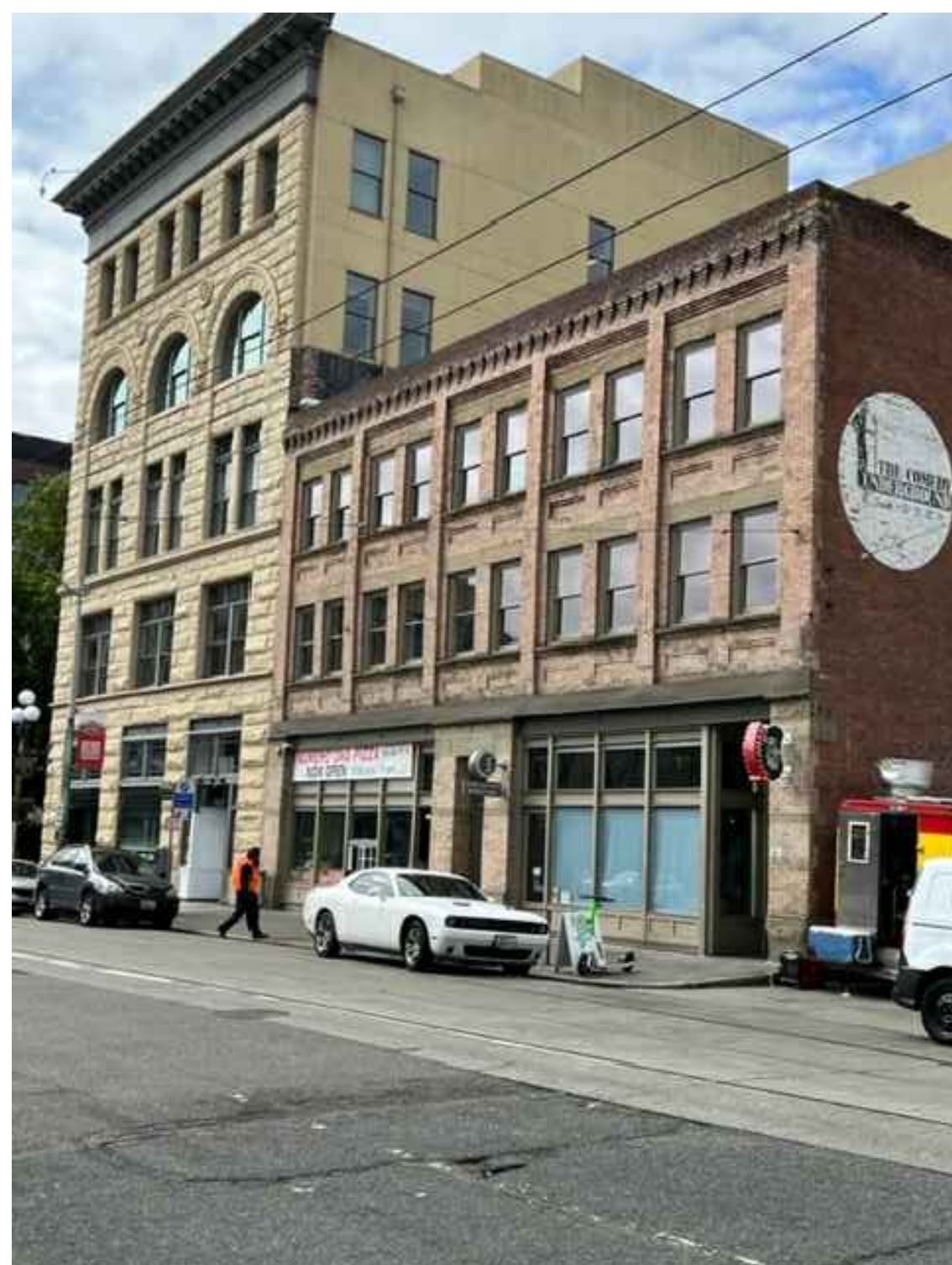
view from southeast, showing existing ground floor signage & entries
